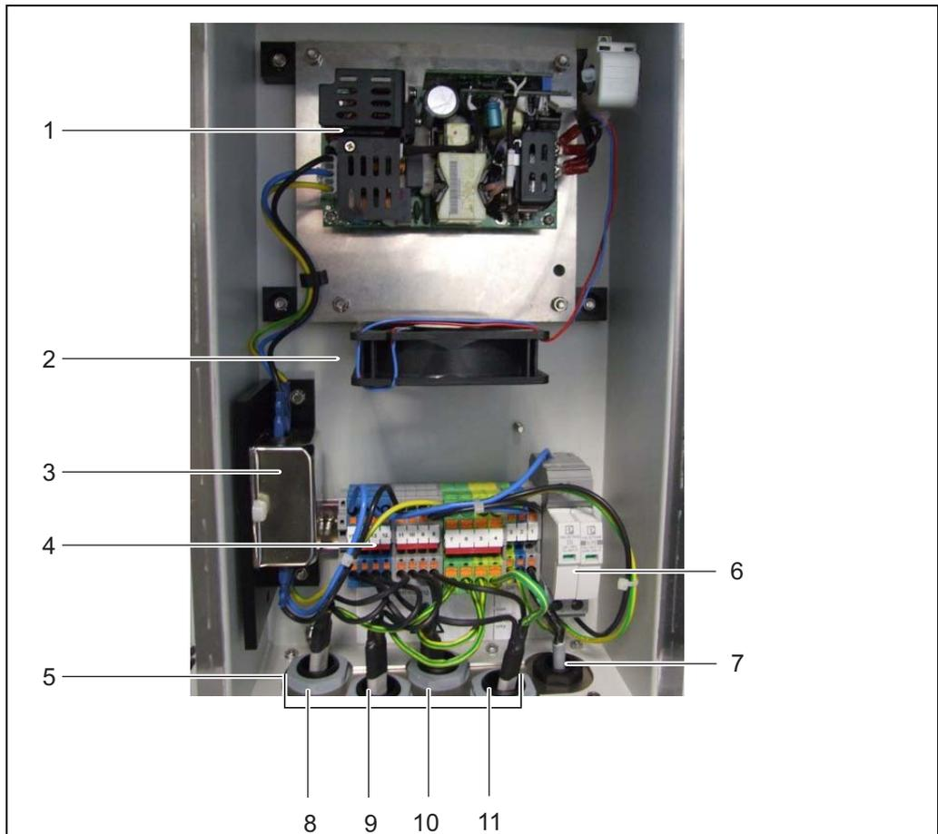
figure 5-18 Connections of the power supply box
